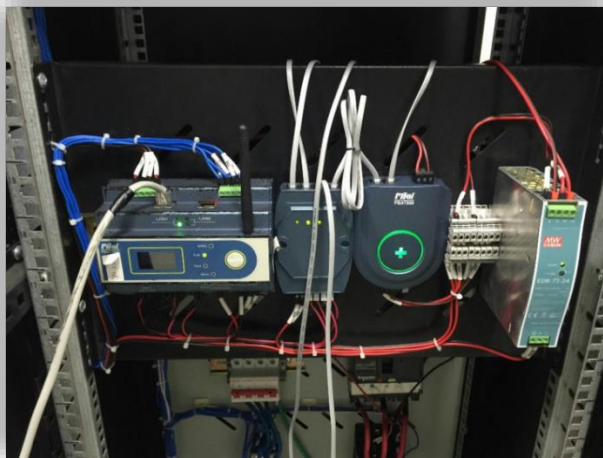
FIGURE 3 GATEWAY, STRING SENSOR AND POWER SUPPLY.
