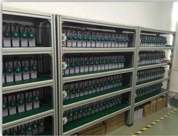
FIGURE 2 BATTERIES WITH SENSORS IN BATTERY BANKS
