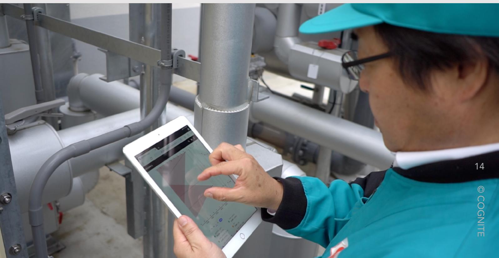
on computers and handheld devices, Operation Support streams data from CDF. By scanning a tag on any piece of equipment in the manufacturing plant, Yokogawa's maintenance workers can now pull up all real-time and historical data, documentation, maintenance records, pictures, and more information relevant to that equipment.
