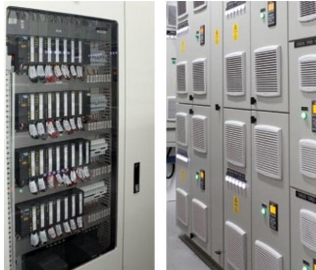
Instrumentation panels enable the remote monitoring and control of the air-conditioning system.
