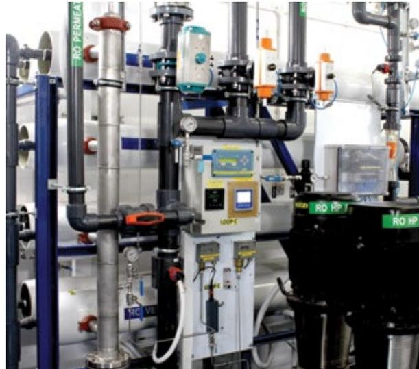
Equipment required for ensuring process water quality include filters (image above) and reverse osmosis high pressure pumps (image below).
