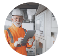
Control Room Operators
