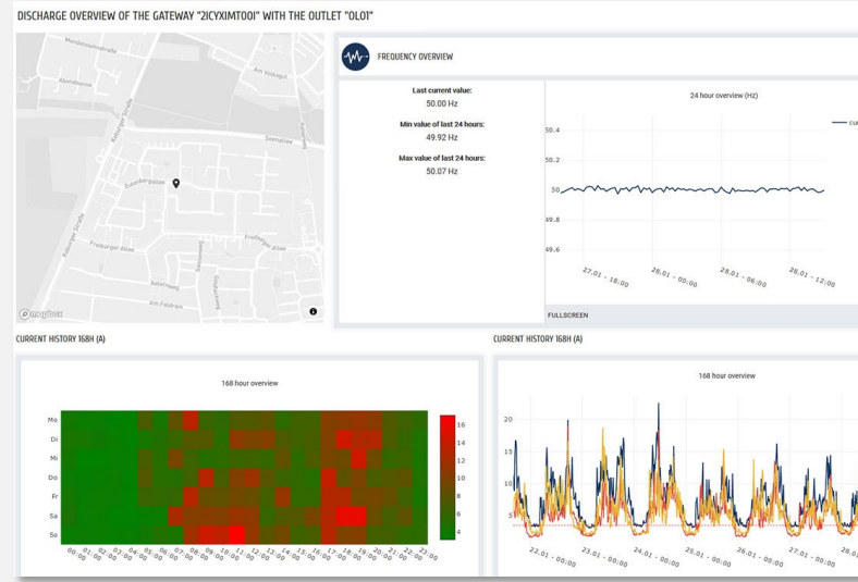
Drill down on transformer and gateway performance with 1x/minute data
