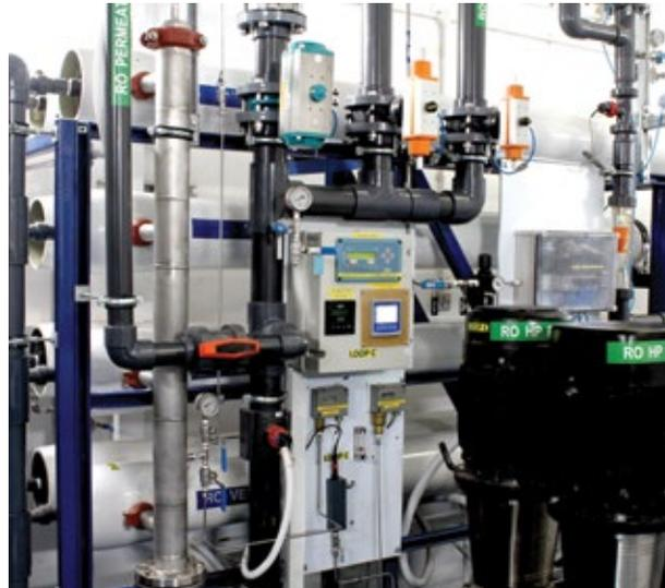
Equipment required for ensuring process water quality include filters (image above) and reverse osmosis high pressure pumps (image below).
