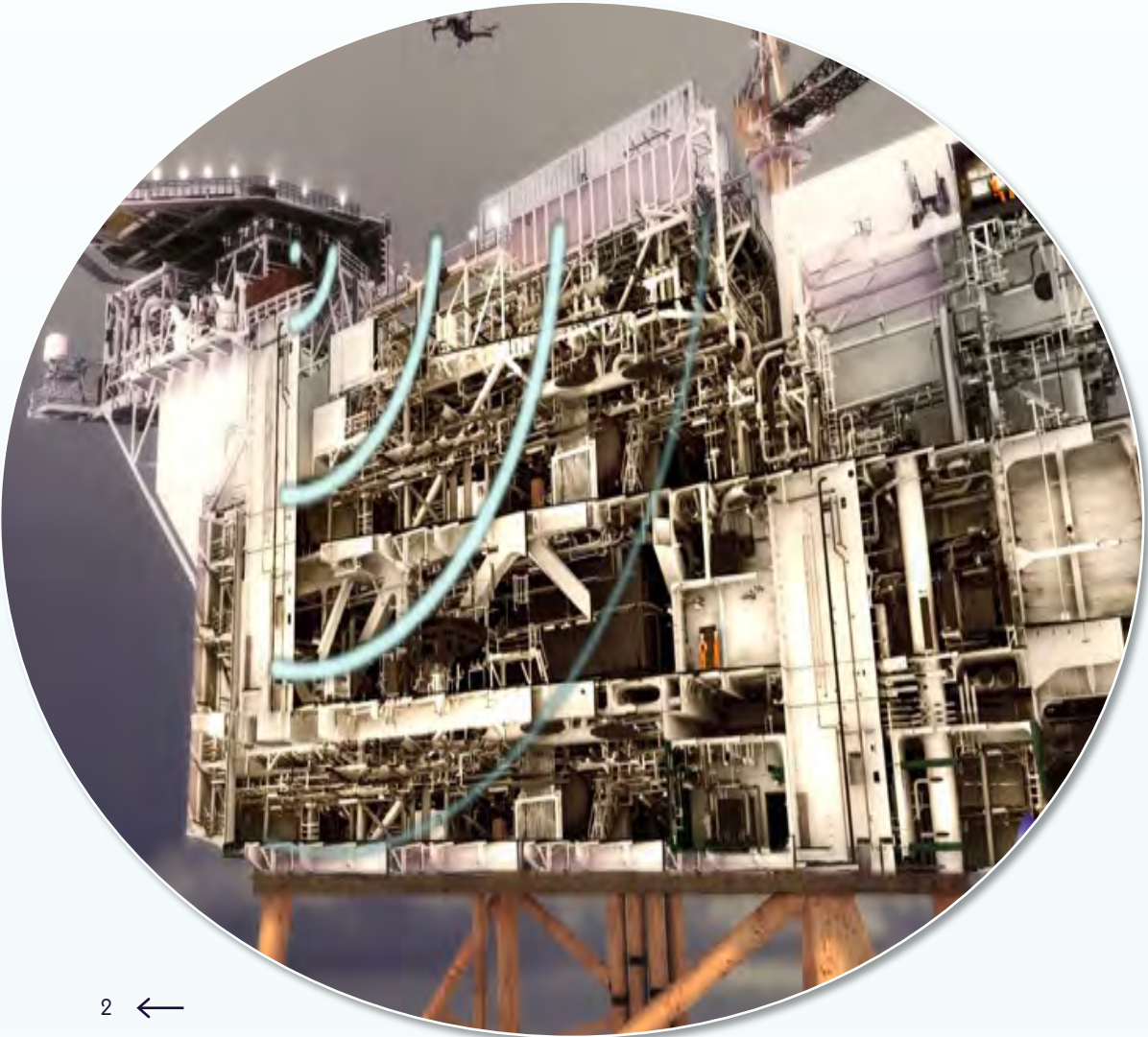
Internal 5G installed
