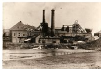
The Colliery Works – Shotton
