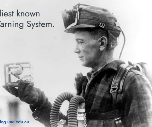
Mining foreman R. Thornburg shows a small cage with a canary used for testing carbon monoxide gas in 1928. (George McCaa, U.S. Bureau of Mines)
