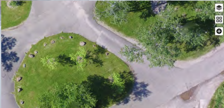
Site Inspection using Orthomosaic maps
