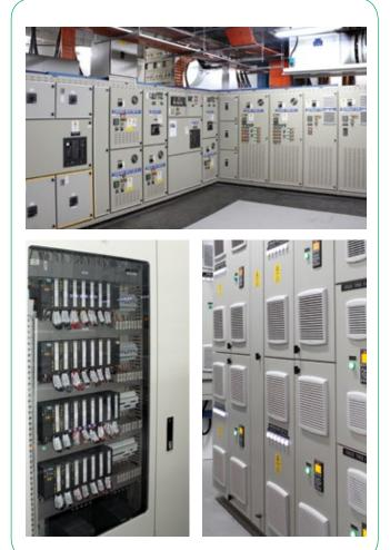
Instrumentation panels enable the remote monitoring and control of the air-conditioning system.
