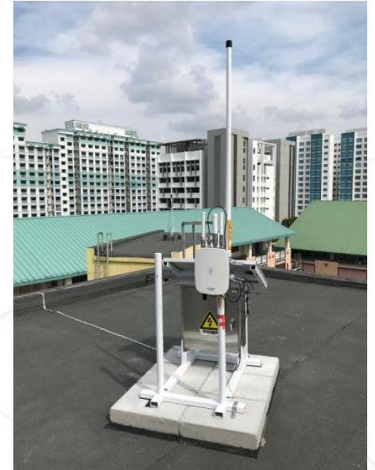
One of our LoRaWAN Outdoor Gateway installed in Jakarta: IP backbone (3G/4G) & Solar Panel with Battery (runs 24hours)
